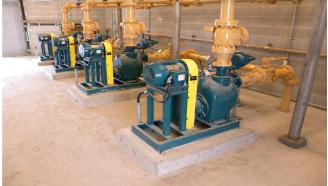
Pump station upgrade With Trash Flow Pumps
