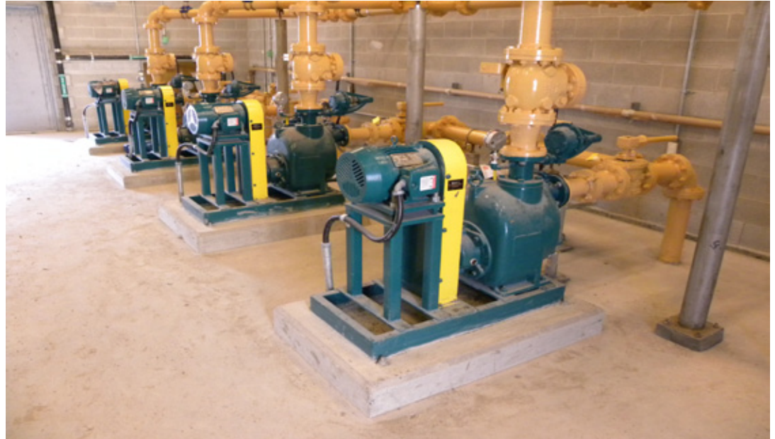
Pump station upgrade With Trash Flow Pumps
